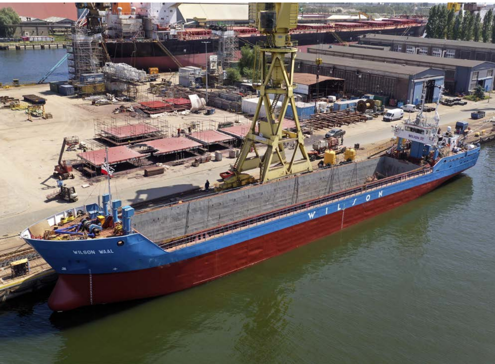
We retrofitted the Wilson Waal with a Ballast Water Treatment System. The vessel's hatch covers were dismantled – here we can see them under repair on the land. Photo: Sławomir Lewandowski
